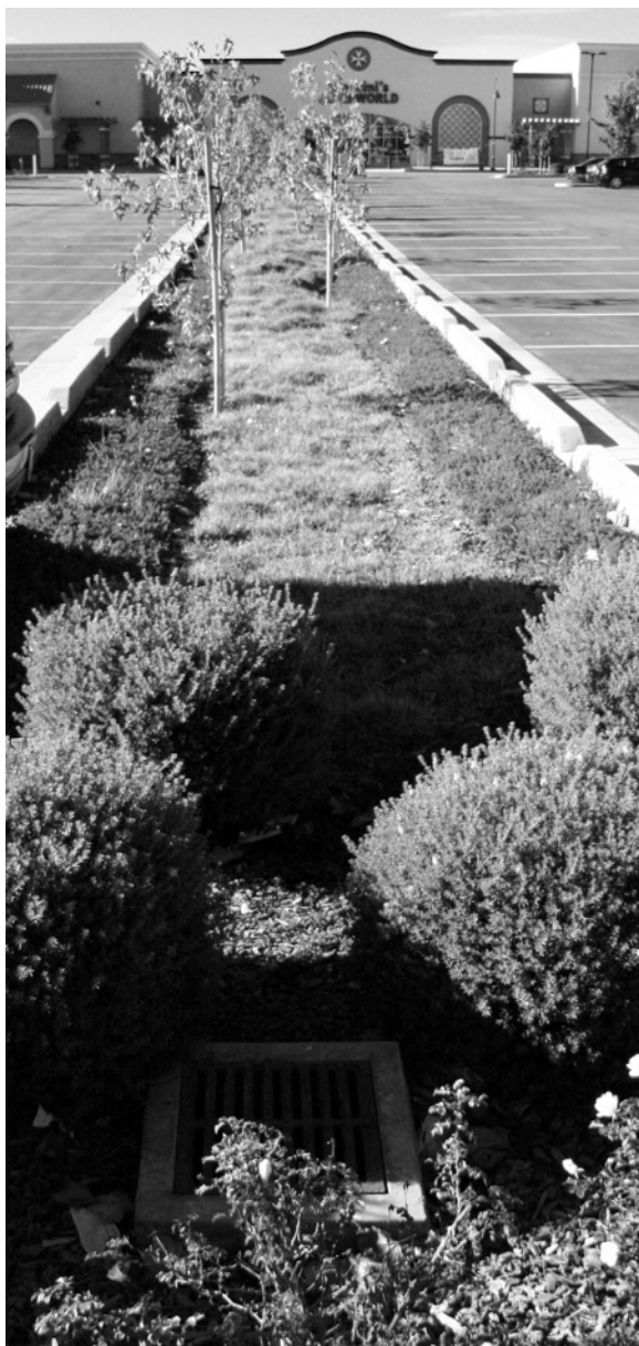
Figure 1: Image of a parking lot bioswale. Inlet (untreated) stormwater samples were collected from several of the curb openings to the bioswale. Outlet (treated) stormwater samples were collected from a drainage pipe located inside an overflow grate located at the top of the image (not shown). Please click here to view a larger version of this figure.
