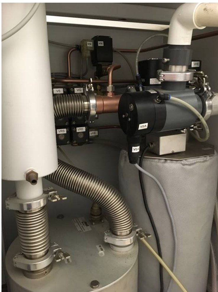
Figure 3. The catalyst container is connected to the main chamber by two valves, which allows the atmosphere to circulate through the catalyst bed.
