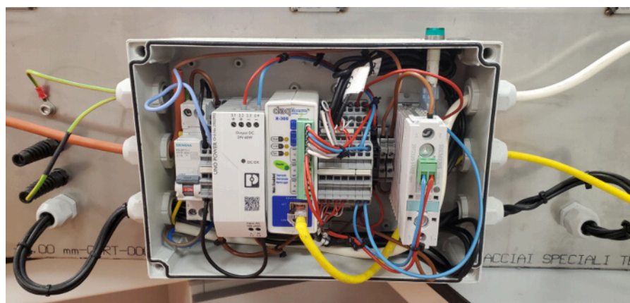
Figure 7: Main junction box of the electronic unit attached to the temperature gradient block. Please click here to view a larger version of this figure.
